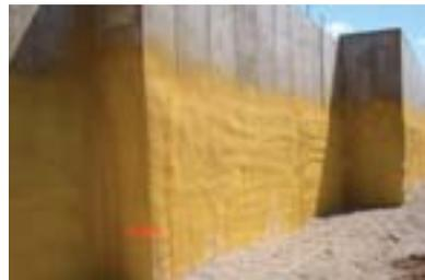
Retaining wall insulation and moisture barrier
