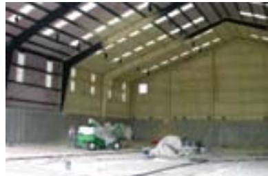
Interior insulation and air barrier
