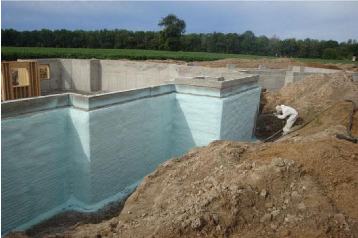
**Figure 3 – Exterior below-grade wall installation (photo)**
