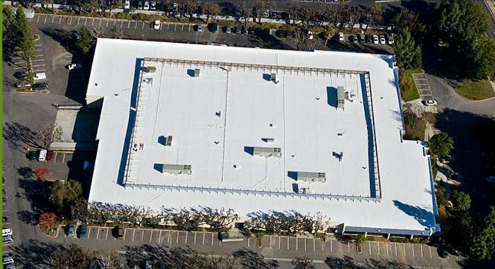
Spray polyurethane foam is the fastest growing insulating product in the world. As a roofing material it provides many benefits over traditional roofing materials. Exceptional durability, unmatched R-value, air barrier properties and a multitude of additional benefits make it a truly versatile roofing system.
