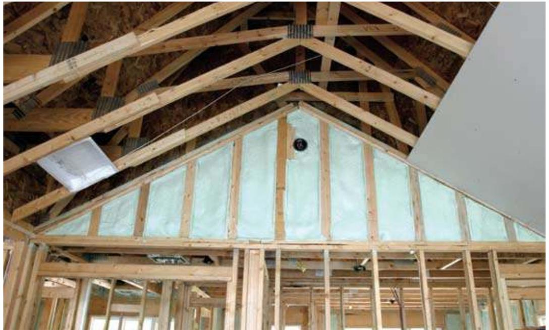
The WALLTITE insulating air barrier system for multi-unit residential, industrial, commercial and institutional buildings is approved by the Air Barrier Association of America (ABAA) to meet or exceed all current State Commercial Energy Codes, and is installed only by approved applicators with third-party quality control inspection.
