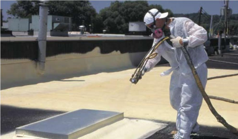
FE 348 SPF is among the most efficient of all roofing insulation materials. In fact, when combined with appropriate coatings, some BASF Polyurethane Foam Enterprises FE 348 systems are ENERGY STAR® approved.
