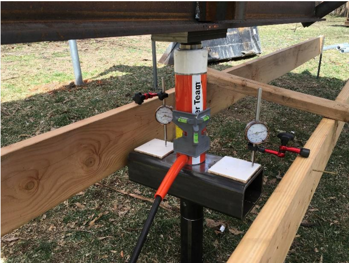
Figure 2: Load test performed on pier in Raytown, MO
