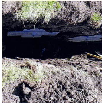
Install Exterior Soil Plate and Nut
