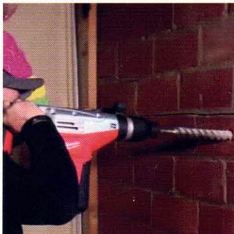
Drill Hole for All Thread In Wall
