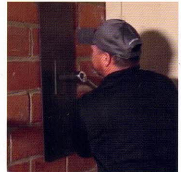
Torque Down Wall Plate and Washer
