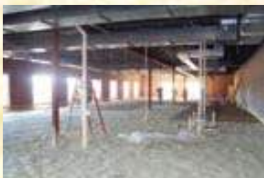
Under slab insulation and moisture barrier
