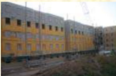
Exterior insulation and air barrier
