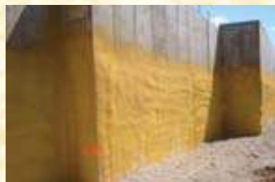
Retaining wall insulation and moisture barrier
