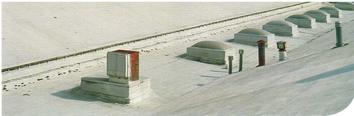
Proven performance: August 1983 Ply System application
