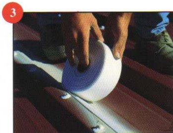
Treating the vertical seams with Spunflex fabric
