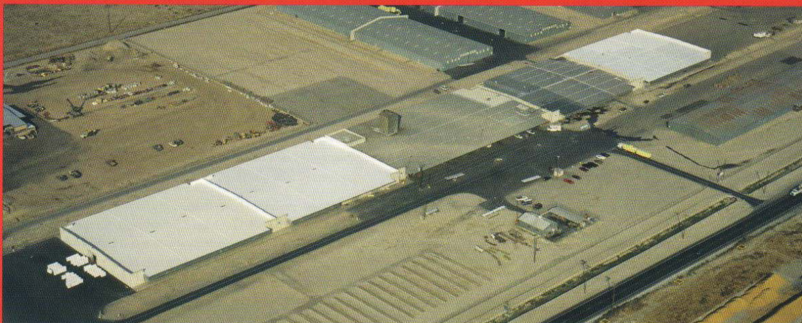
Warehouse storage facility, California — 250,000 sq. ft.
