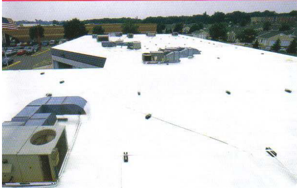
After foam roofing systems
