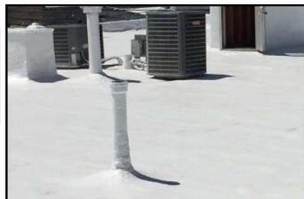
**MINIMIZES THERMAL SHOCK**—Because a polyurethane foam roofing system is seamless, has a high R-value and is covered by a reflective elastomeric coating, it greatly reduces the thermal shock a building is subjected to because of fluctuating outdoor temperatures.
