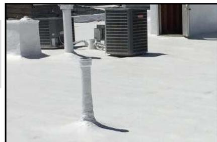
**MINIMIZES THERMAL SHOCK**—Because a polyurethane foam roofing system is seamless, has a high R-value and is covered by a reflective elastomeric coating, it greatly reduces the thermal shock a building is subjected to because of fluctuating outdoor temperatures.
