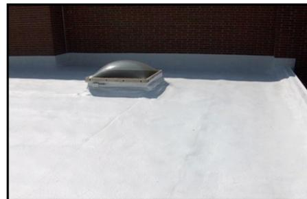
**ELIMINATES WATER PONDING**—When re-roofing, ponding water can be eliminated by adding increased thickness of polyurethane foam in low areas. Building up these areas and sloping the roof so that it drains properly will eliminate ponding water and reduce the load factor on the roof caused by water accumulation.
